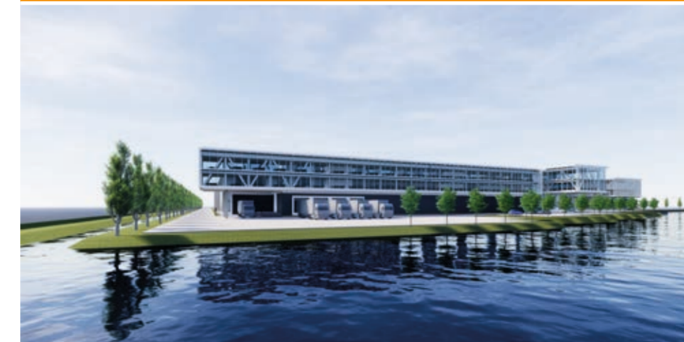
Lely F2, Maassluis, NL Architect: ConverseArchitects
