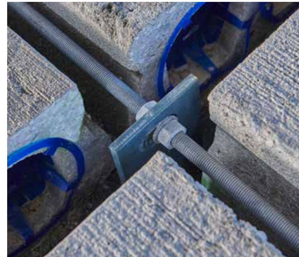
VBI project Phoenix in Zevenaar (detail)
